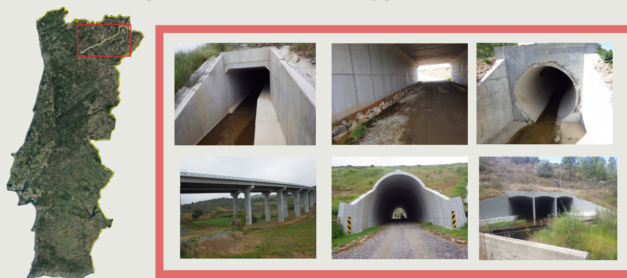
Fig 1. A4 motorway location (Google Earth) and underpasses of different types.
