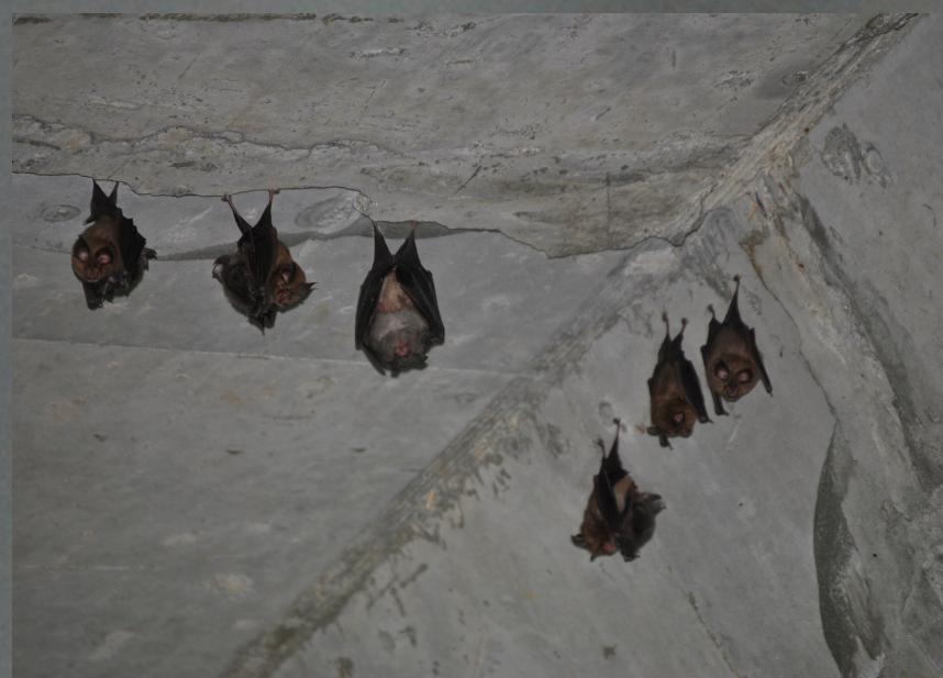
Fig 3. Breeding colony of the Rhinolophus hipposideros in a viaduct box girder.
